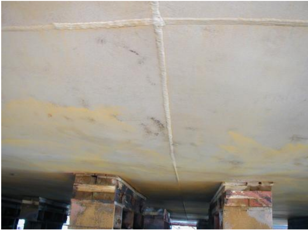
Photo 15. LINDA KOSAN underwater part – surface preparation.
