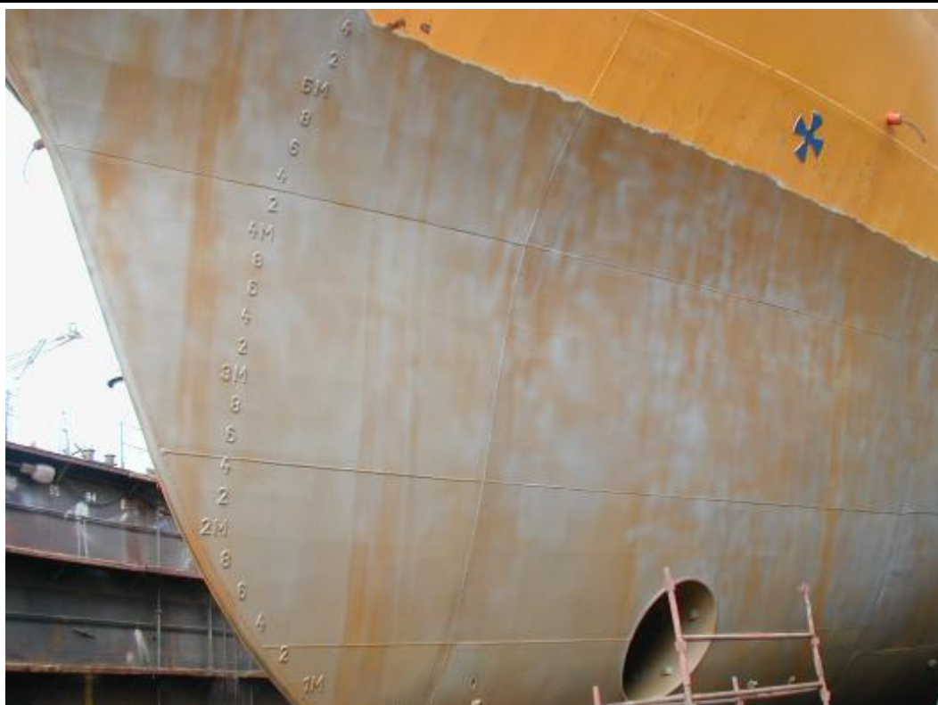
Photo 13. LINDA KOSAN underwater part – surface preparation.
