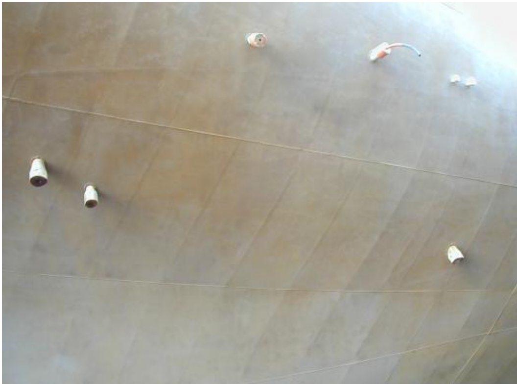
Photo 10. LINDA KOSAN underwater part – surface preparation.
