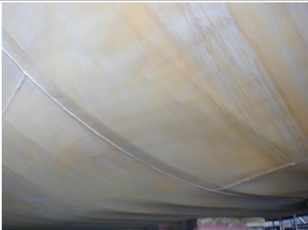
Photo 2. LAURA KOSAN underwater part – surface preparation.
