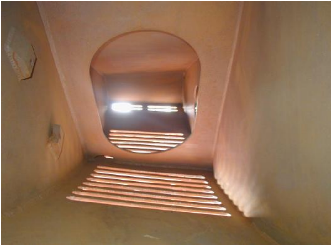
Photo 16. LINDA KOSAN underwater part sea chest – surface preparation.
