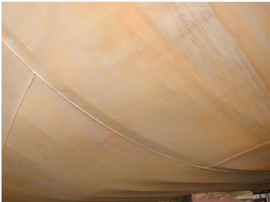
Photo 3. LAURA KOSAN underwater part – surface preparation.
