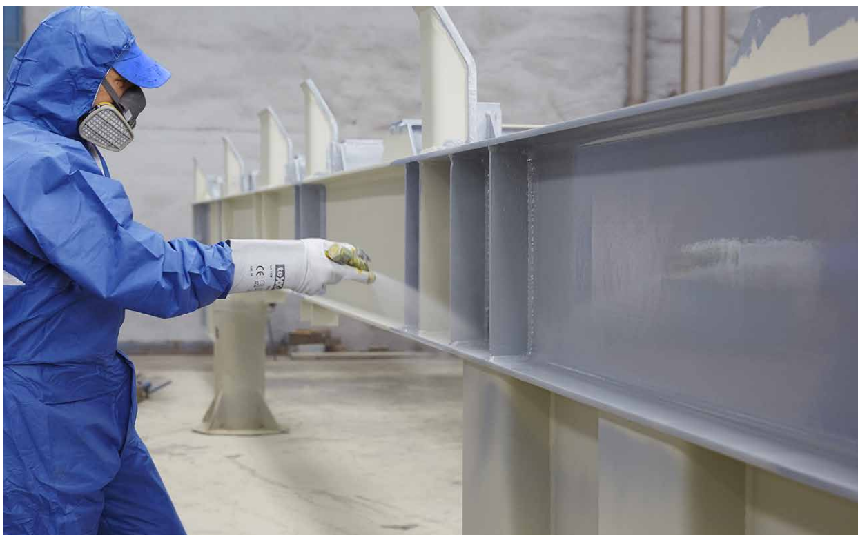
Production and coating of steelwork for docks, Szczecin, Poland
